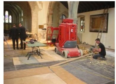
Scissor lifts permissible to 2 tonnes with additional layer of 2 x 18mm ply.
