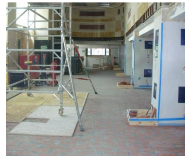
Towers and scaffold should be erected on 1 x 18mm ply sheet
