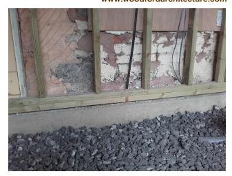
As an alternative to a conventional slab TechnoPor Glass Foam was used. Adopting this method of construction forms a strong and insulated base without the drying out time of a concrete slab.
