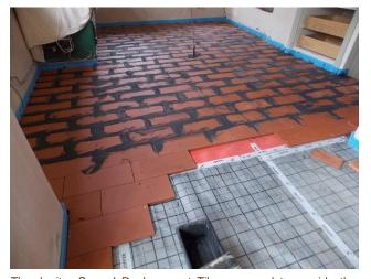
The Jupiter Screed Replacement Tile was used to provide the ideal substrate for the large-format finished floor tiles. The SRT system decouples the finished floor and allows Jupiter to guarantee finished floor tiles against failure for five years.
