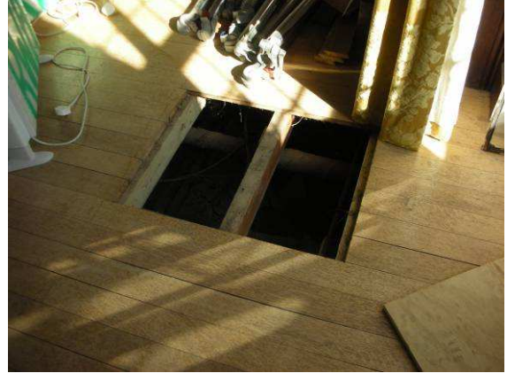
Existing suspended wooden floor removed to expose joists
