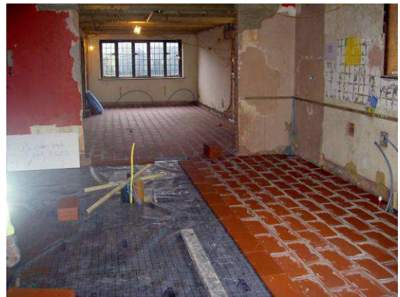
20mm thick Screed Replacement Tiles installed directly over the existing floor joists on JUPITER System foil.
