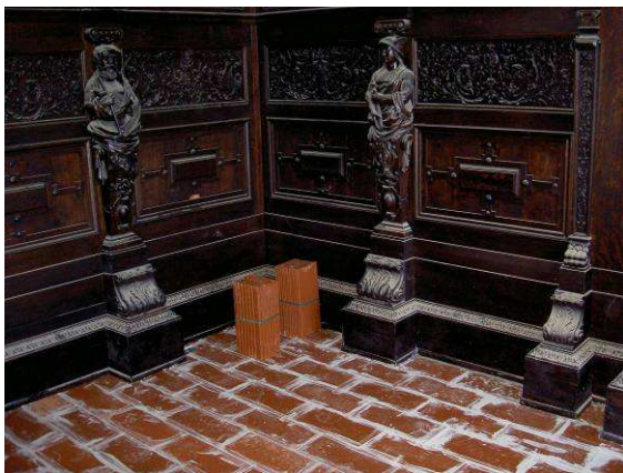
After 36 hours S.R.T. substrate ready to accept finished floor.
