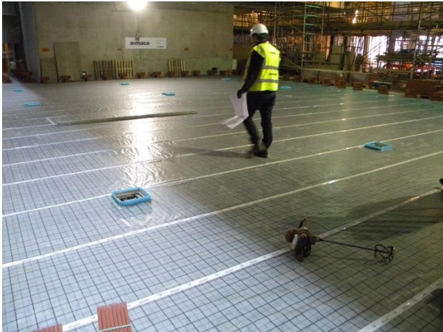
JUPITER system foil is laid on top of the Ideal EPS heating panels as a slip membrane prior to the laying of the Screed Replacement Tile system
