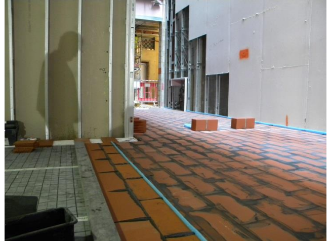
The JUPITER SRT system is laid forming the perfect substrate for stone and tile floor finishes of any size and thickness
