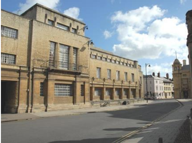
The Weston Library, designed by Sir Giles Gilbert Scott and constructed in the 1930s
