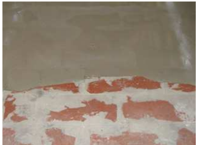
After 24 hours SRT's are set. filling compound such as Thomsit RS 88 is applied to ensure that any discrepancies do not show through the finished floor.
