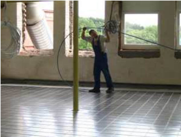
Laying the JUPITER pipe in the Jupiter IDEAL panels
