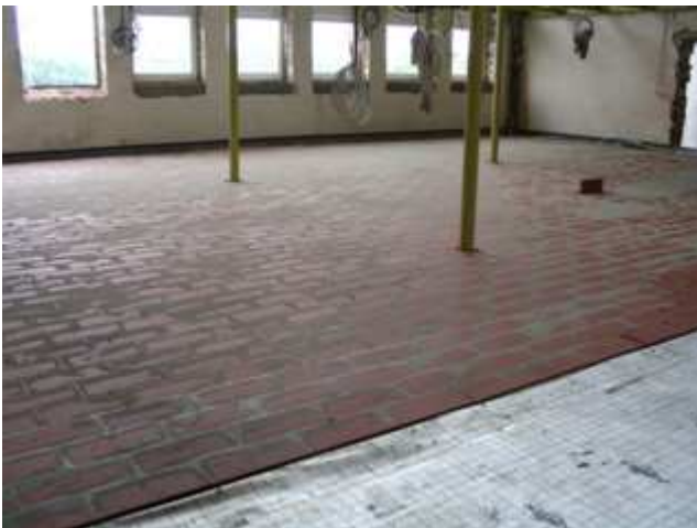
Up to 400m 2 of Screed Replacement Tiles can be laid without the need for expansion gaps.
