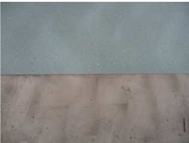
The linoleum is laid on the cured smoothing compound.
