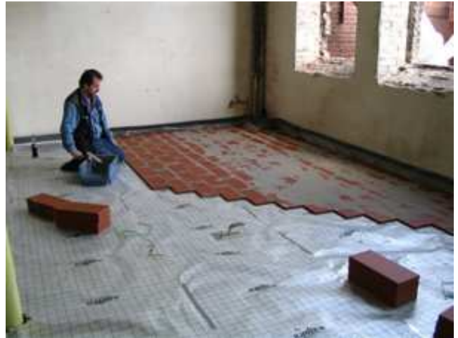
Screed Replacement Tiles are glued together in brick bond format on the JUPIETR system foil.
