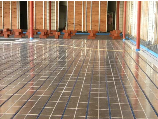
The primary insulation and underfloor heating panels were installed within 1 week.
