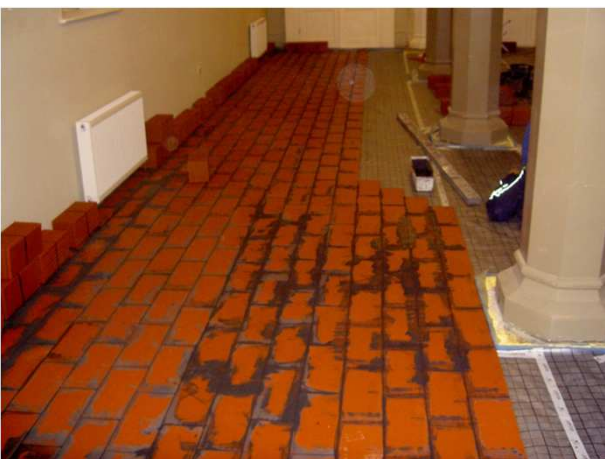
Screed Replacement Tiles installed in brick bond format .
