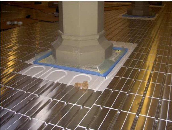
JUPITER IDEAL system (125mm pipe centres) installed throughout.
