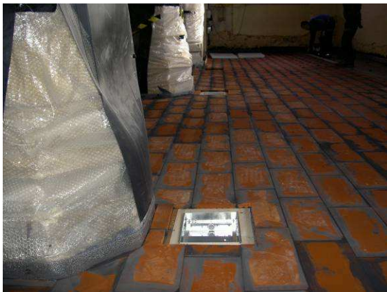
The JUPITER Screed Replacement Tile is installed over the IDEAL heating elements acting as a substitute to screed.
