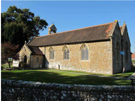
St Peters & St Pauls church in Ashington is the second church in which the JUPITER IDEAL system with Screed Replacement Tile was specified.
