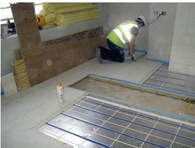
Fermacell flooring elements being installed using glue and diverging staples.
