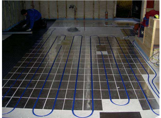
IDEAL EPS installed over Kingspan K3
