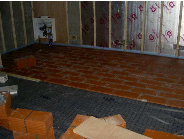
Screed Replacement Tiles used installed as substrate for resin floor
